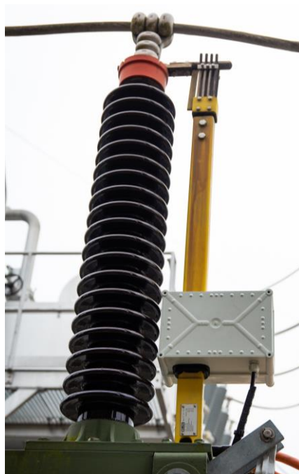
Figure 13: Neutral point measurement system - Mounted type
