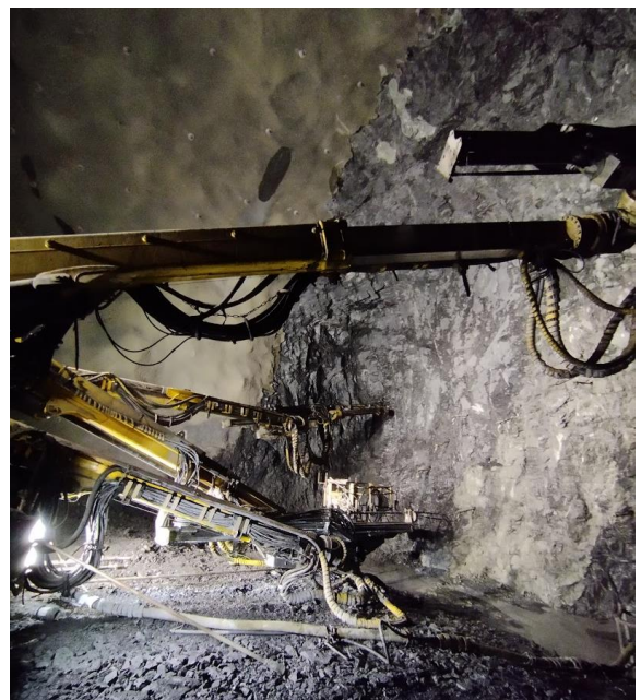
Figure: Unsupported full face excavation in Norwegian hard rock conditions.
